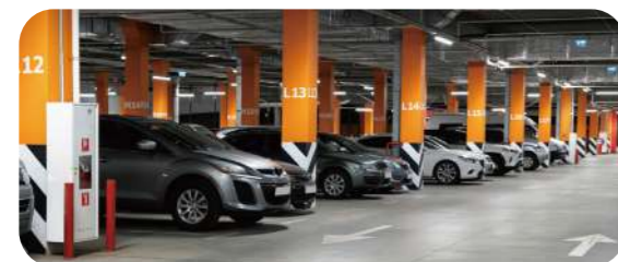
Smart Parking Lot
