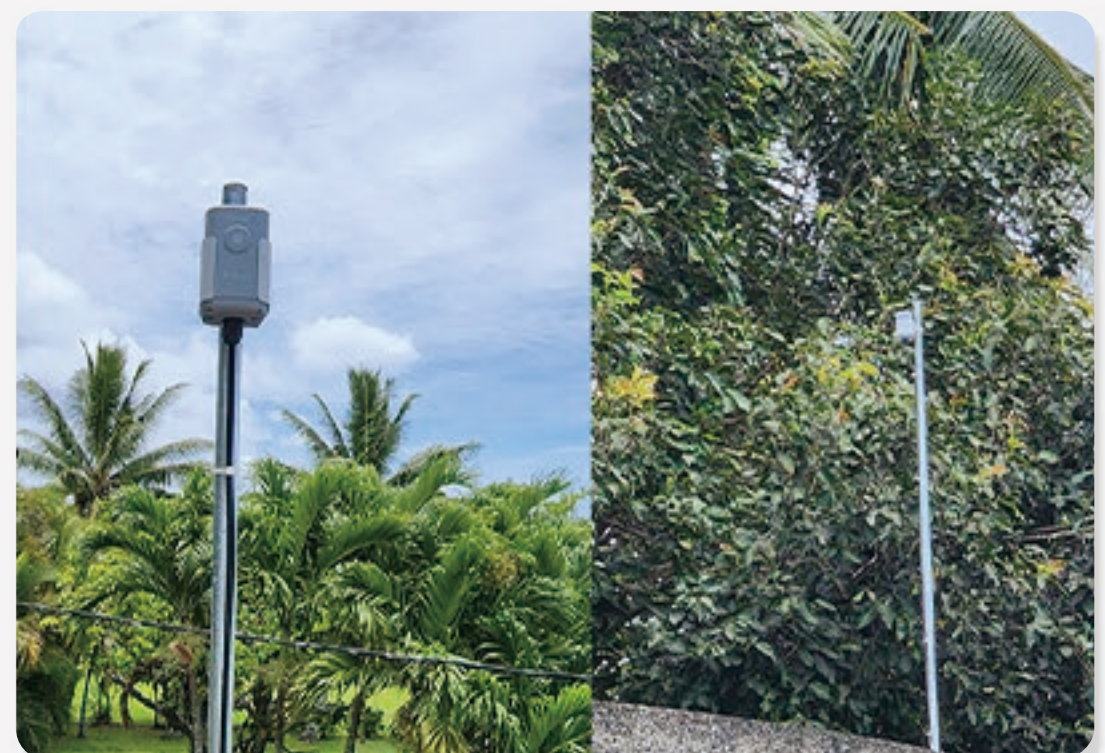
Picture 6 Project Deployment
