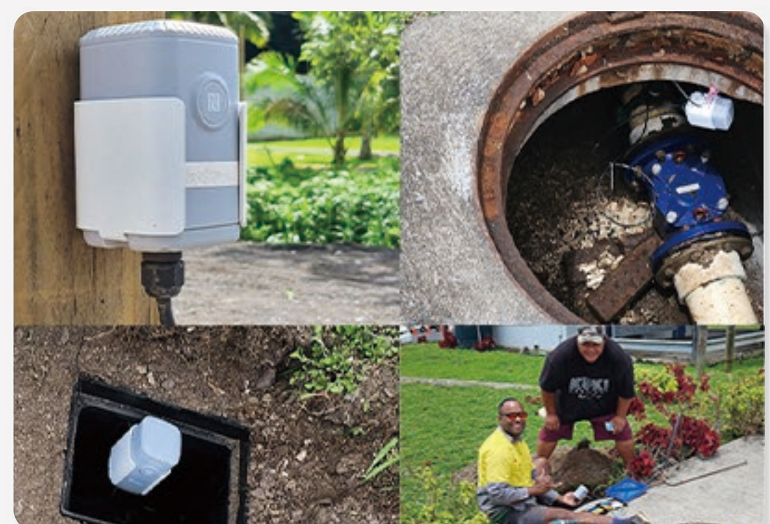
Picture 7 Project Deployment
