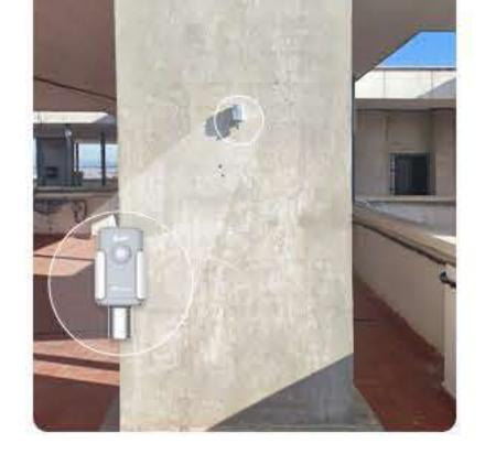
The Ebento project employs advanced IoT solutions from Milesight to monitor and analyze the performance of newly implemented insulation technologies. 48 AM103L 3-in-1 IAQ Sensor and 4 EM500-CO<sub>2</sub> Outdoor CO<sub>2</sub> Sensor are strategically placed to collect data on thermal efficiency, which is crucial for assessing the effectiveness of the insulation under various environmental conditions.
