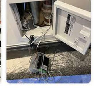
A UG56 Industrial LoRaWAN® Gateway or a UG65 Indoor LoRaWAN® Gateway is installed every two floors in the garbage chute rooms ceiling, connected to a dedicated building VLAN. Additionally, a UG67 Outdoor LoRaWAN Gateway is located at the top of the building, acting as a master (in fleet mode) and providing a backup cellular connection to the Internet. Each Milesight controller and gateway is connected to the generator, ensuring they remain active in case of a power failure.
