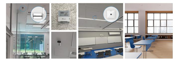
Milesight VS121 AI Workplace Occupancy Sensor detects real-time presence with up to 95% accuracy. Combined with IAQ sensors, the data is transmitted via LoRaWAN® to BMS platforms through BACnet/IP. This enables automated ventilation adjustment, smart room release, and full environmental visibility-creating a responsive and efficient smart campus environment without requiring major system overhauls.
