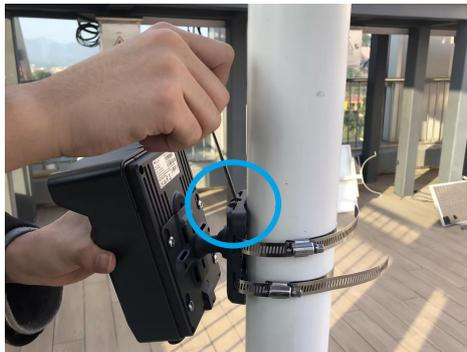
**! Note:** The bracket fixation at this point is only to temporarily secure the camera at a reasonably suitable angle. The final fixation angle should be adjusted based on the image results.
