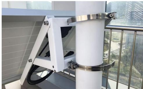
3. Securely fix the bracket at a height of **2 to 4 meters (16mm lens)/2.5 to 3 meters (6mm lens)**, with a recommended height of 3 meters, ensuring correct orientation and a sturdy fixation.
