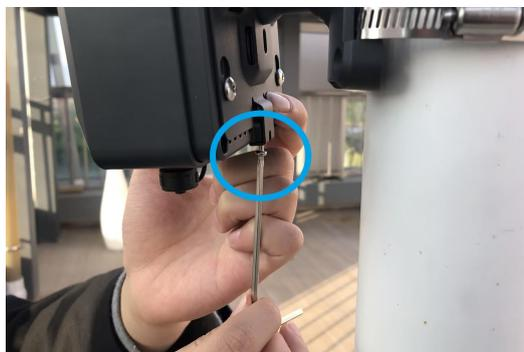
6. You can adjust the angle of the bracket by tightening or loosening the screws at the top. Please ensure that the angle and direction are approximately aligned.
